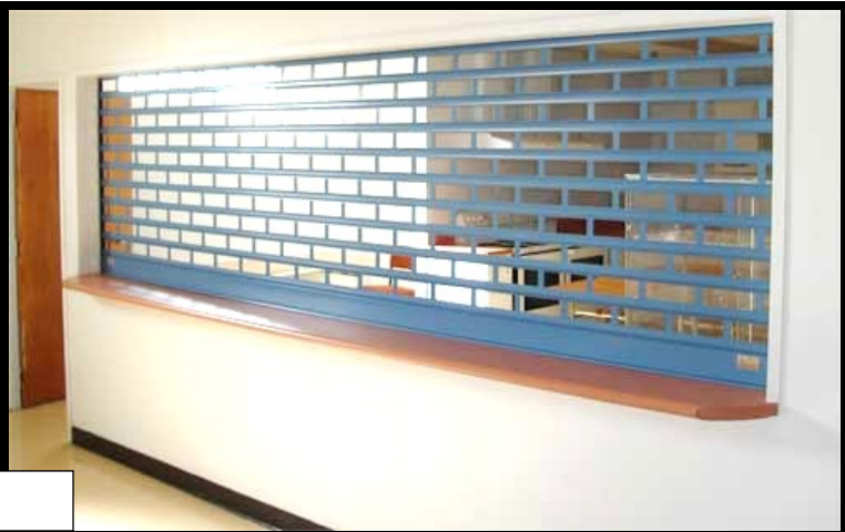
Grill type Roller Shutter Doors with Tubular Motor – SOMFY brand – 5 Years Manufacturer Warranty with manual cranking System
